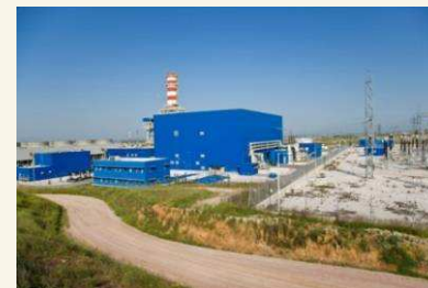
Thessaloniki power plant
